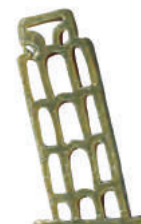
#609/04 Leaning Tower of Pisa
