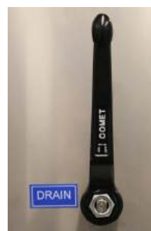
Vertical = Drain Open
