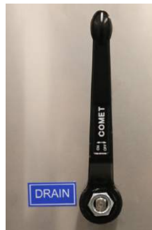
Vertical = Drain Open
